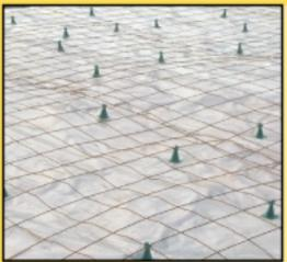
When Valor is pouring a slab it's IMPORTANT to make sure that mesh-ups are installed so that the wire is NOT being pushed down.
