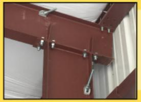
Valor rafters are bolted down to the **TOP** of the column, creating a stronger connection.
