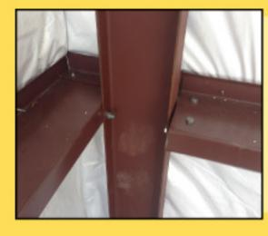
Where the purlin stops at the corner column, Valor Steel Buildings puts a sheeting angle in the corner so that the panel is COMPLETELY screwed off.
