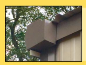
Valor uses a corner box that **CLOSES** up the gable/rake trim. This helps prevent birds from nesting. Gutters can also be installed.
