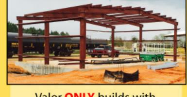
Valor ONLY builds with structural I-BEAMS, which is the best & strongest framing. Tapered systems are weaker plates, half-welded, to form a cheaper system with less steel.
