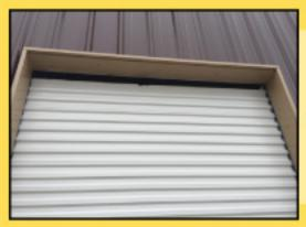
Valor installs a brush guard to close the gap at the top of the roll-up door. This helps to **PREVENT** birds & insects from entering.
