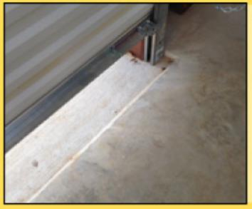
Valor forms a notch out in the concrete so the roll-up door can sit down **BELOW** the top of the concrete. This helps prevent water & insects from entering your building.
